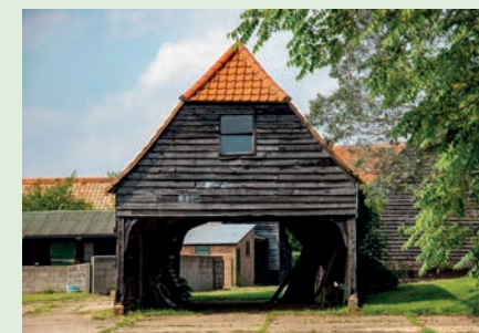
Cart Lodge, Easthorpe Road, Easthorpe
