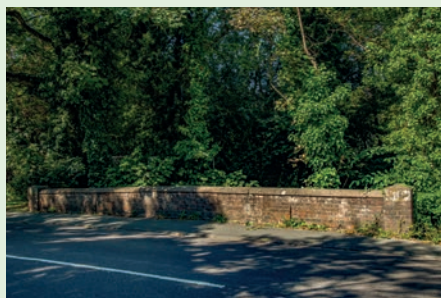
Stanway Bridge, London Road, Copford
