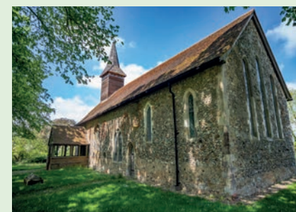
Easthorpe Church, Easthorpe Road, Easthorpe
