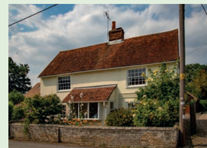
Bell House, Easthorpe Road, Easthorpe
